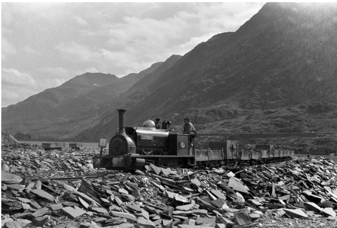
'MAID MARIAN' (HE 822/1903) with engine crew Jack Thomas and Glyn Jones, returning with empty slate waste wagons having just been tipped into Llyn Peris in the background, on Hafod Owen (Ground) level, with the engine guised in her 'original' condition with the brass domed water tank, although the frames were those of stablemate 'KING OF THE SCARLETS' following the 1928 identity swap. August 1949 Photograph by G Shuttleworth/MLS Collection
